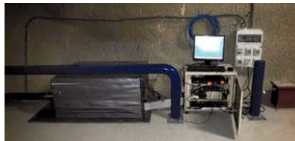
Figure 10.6: New setup of the GAL16 main plinth
