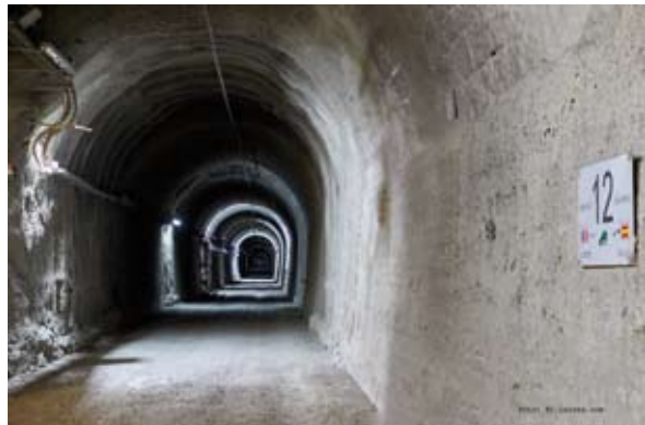
Fig. 1.2: The Train Tunnel at LSC
