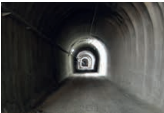
Fig. 1.2: The Train Tunnel at LSC
