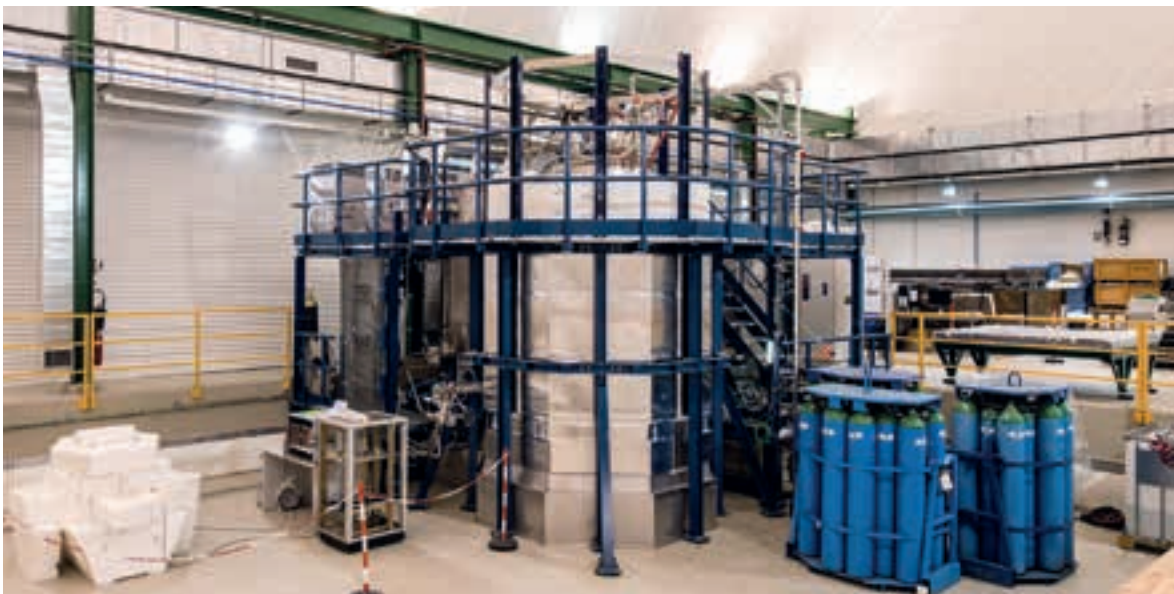
Fig. 5.1 Construction of the ArDM setup for the first phase of the Experiment was completed in underground Hall A of LSC. The polyethylene neutron shield (white, in the centre) was fully constructed to enclose entirely the detector vessel. The lower half was covered with fire protection panels consisting of aluminium sheets (outside) and thermal insulators (inside).
