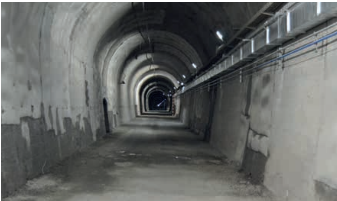
Fig. 1.2 The Train Tunnel at LSC
