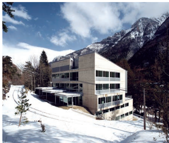
Fig. 4.9. The service building on the surface
